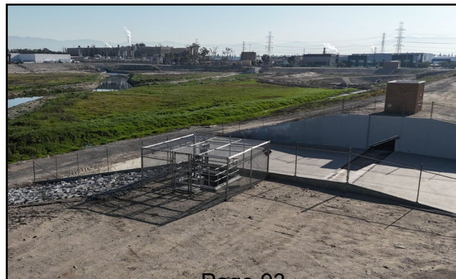
Outlet Control Gate/Rubber Dam System
